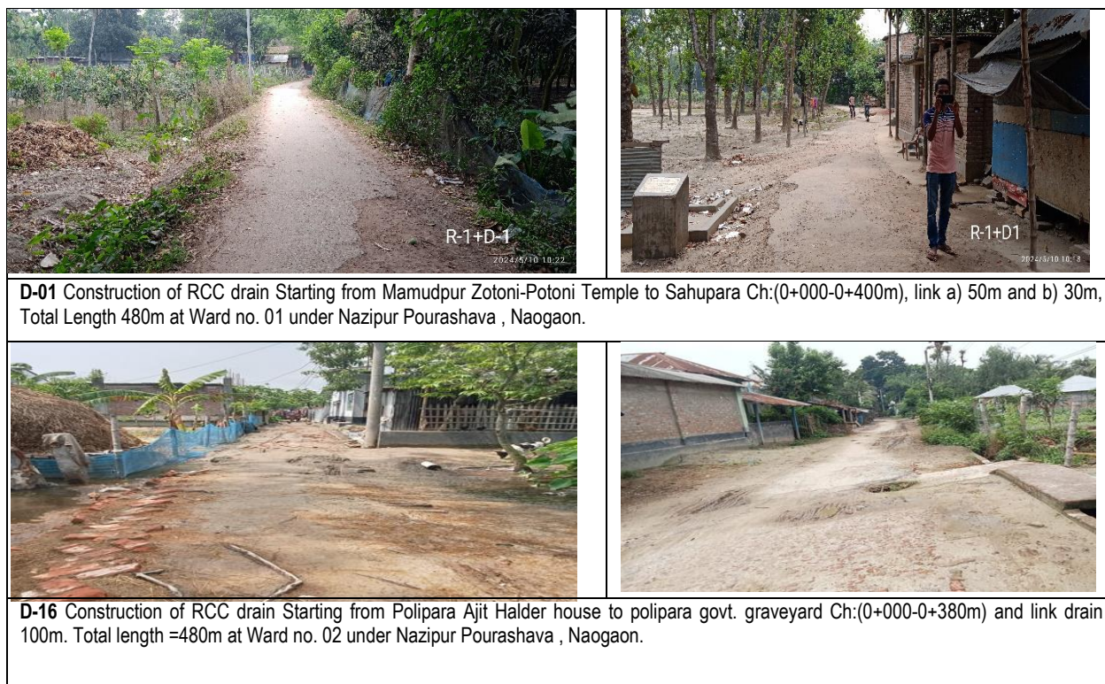
Figure 4:Existing Roads and Drains Picture
